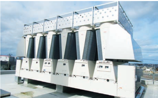
Air-cooled heat pump chiller introduced as part of our ESCO service (heat source equipment for ventilation)
