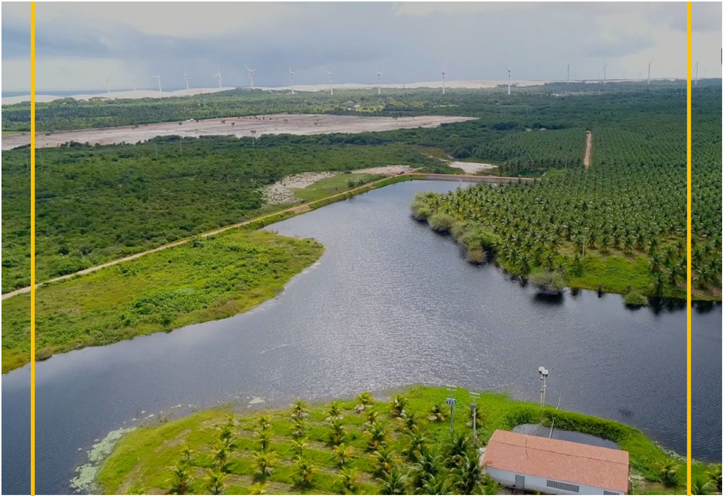
Our eco-dam has a capacity of 7, 834,000 cubic meters.
