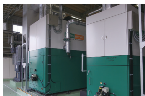
Wood biomass boiler
