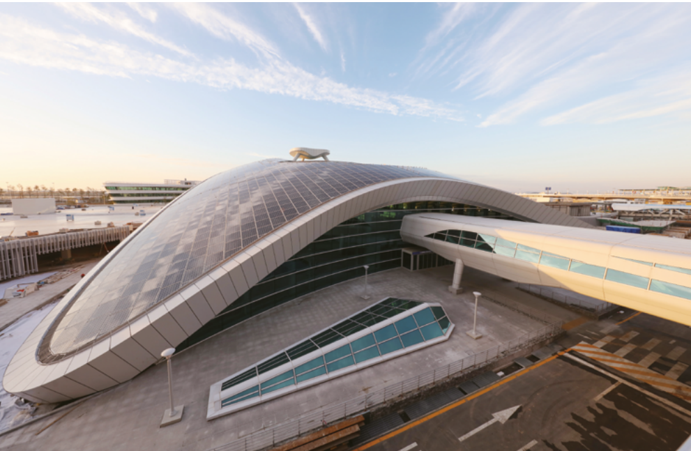
Frontal Exterior Solar Panel Roof in T2
