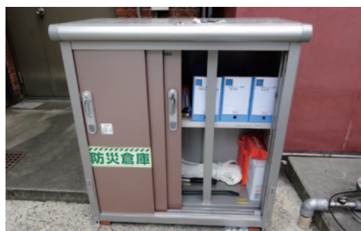
Outdoor emergency cabinet installed
