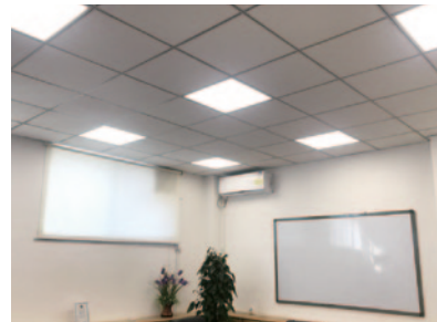
Shifting to LED lighting fixtures
