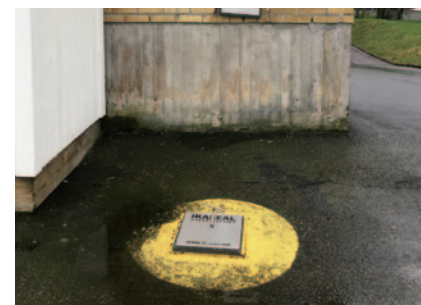
Cover for prevention of effluent leakage
