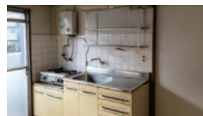
Remodeling (before renovation)
