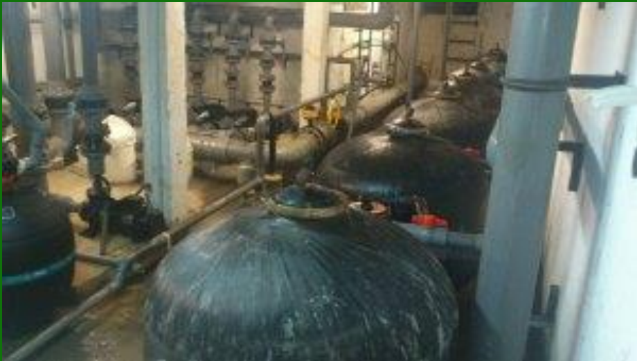
Swimming pool sand filtration Our pool does not use conventional chlorine treatment but various filtration and purification steps
