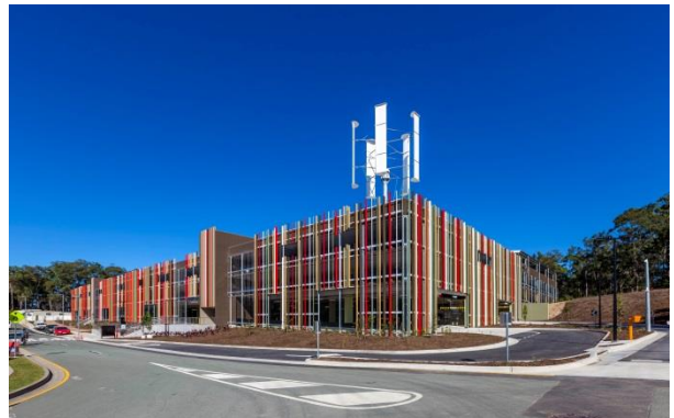
Aquatic Centre features 90kW solar array and green roof and Multi-storey carpark features 100kW solar array and 10kW wind turbine Gold Coast campus
