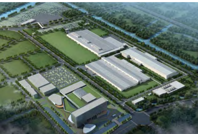
A bird's-eye view of the site of Shanghai GM's new Cadillac plant and PATAc's new R&D facility.
