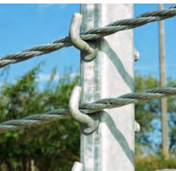
Highway metal barrier that allows for more pliant crash impact.
