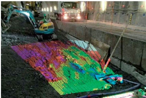
Imaging data projected on the floor of an invert
