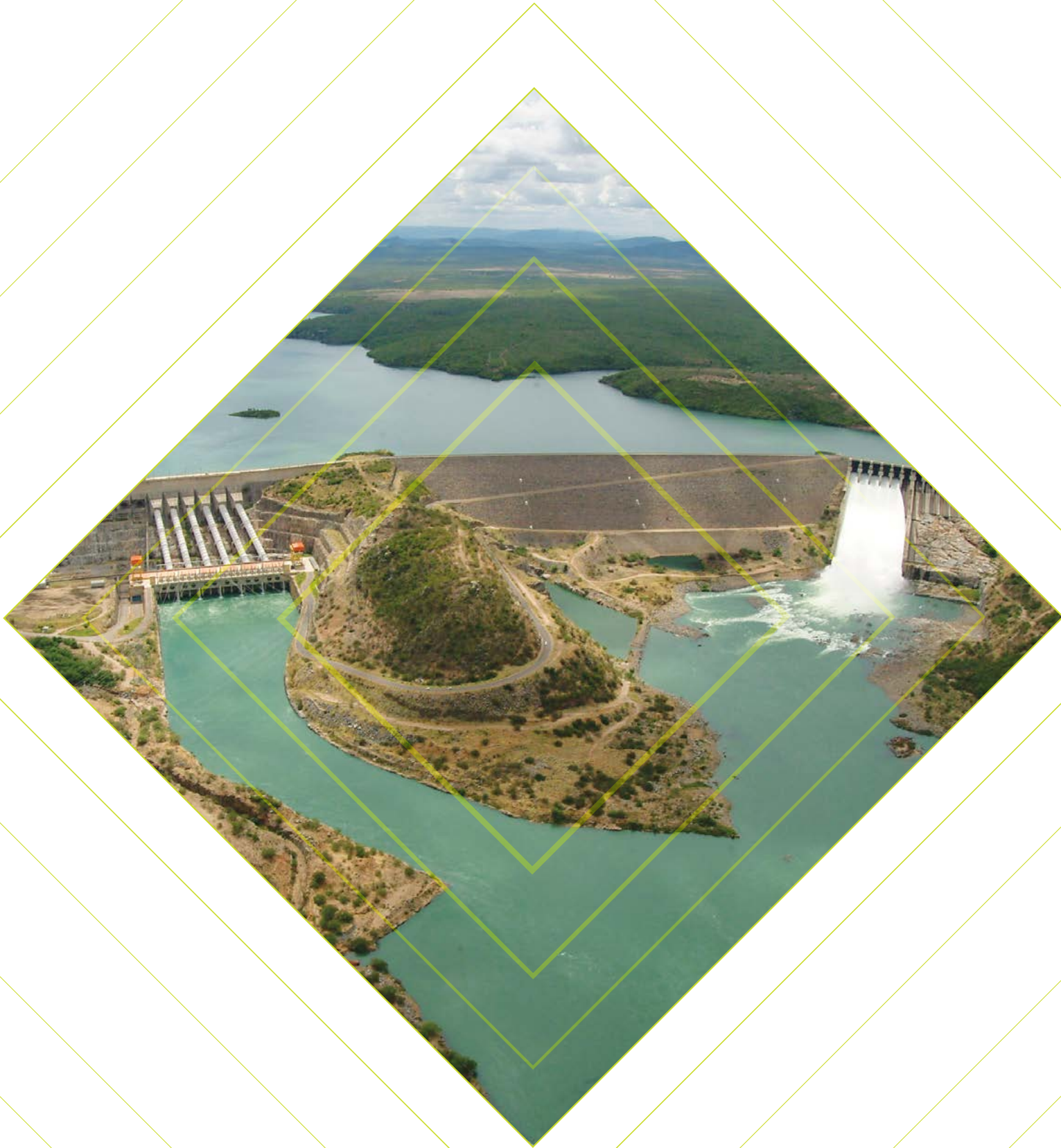
XINGÓ HYDROELECTRIC POWER PLANT
