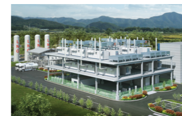
Fuel cell power plant in the frozen logistics complex at Pyeongtaek Oseong
