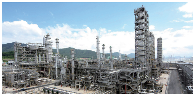
View of the VGO FCC (Vacuum Gas Oil Fluidized Catalytic Cracking Unit) at the Yeosu Complex
