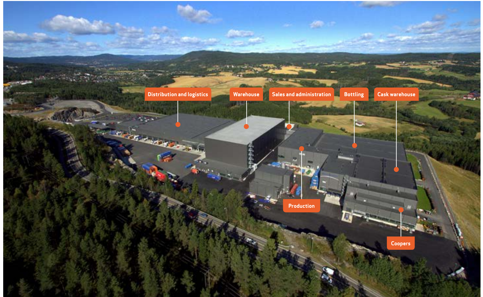
Arcus' production facility outside Oslo, inaugurated in 2012, is as large as six soccer pitches.
