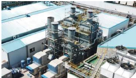
Co-generation Plant at the Ulsan Plant
