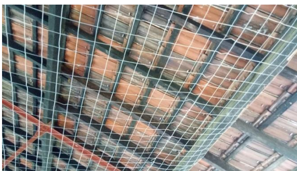
Wire mesh to prevent Pigeons from coming back The Building after the renovation ready for occupation
