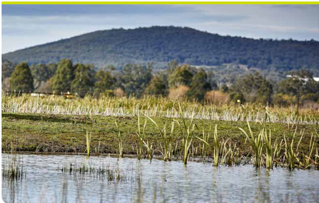
IMAGE: Upper Yarra Sewage Treatment Plant located in the Yarra Valley
