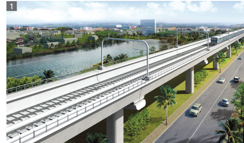
1 HCMC Urban Railroad Line 1 Zone 2 (Vietnam) Project Period: July 2012 – Dec. 2019 Order: KRW 402.8 Billion
