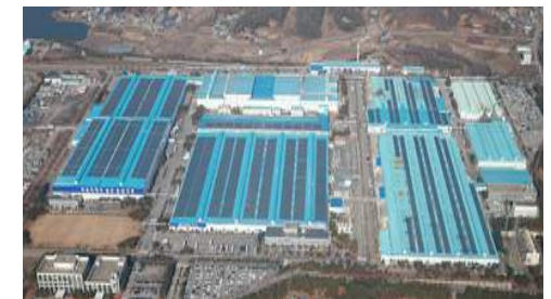
PV power generation facility at the Asan Plant
