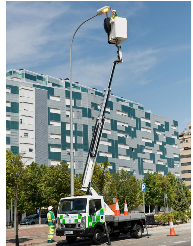
Lighting Maintenance in Madrid.
