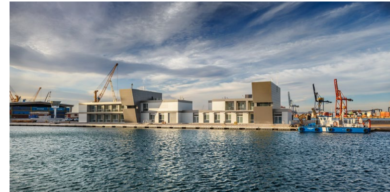
Port Nautical Services Buildings Valencia (Spain).
