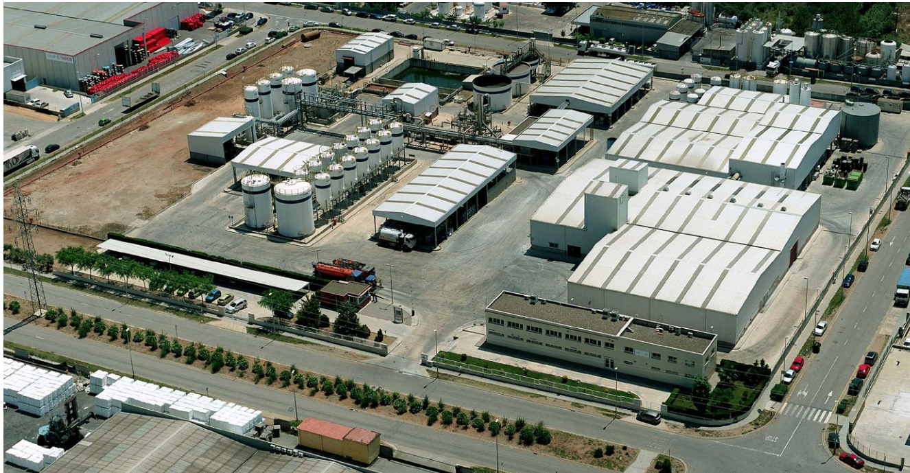
TRISA. Physical and chemical industrial waste processing plant (Tarragona).
