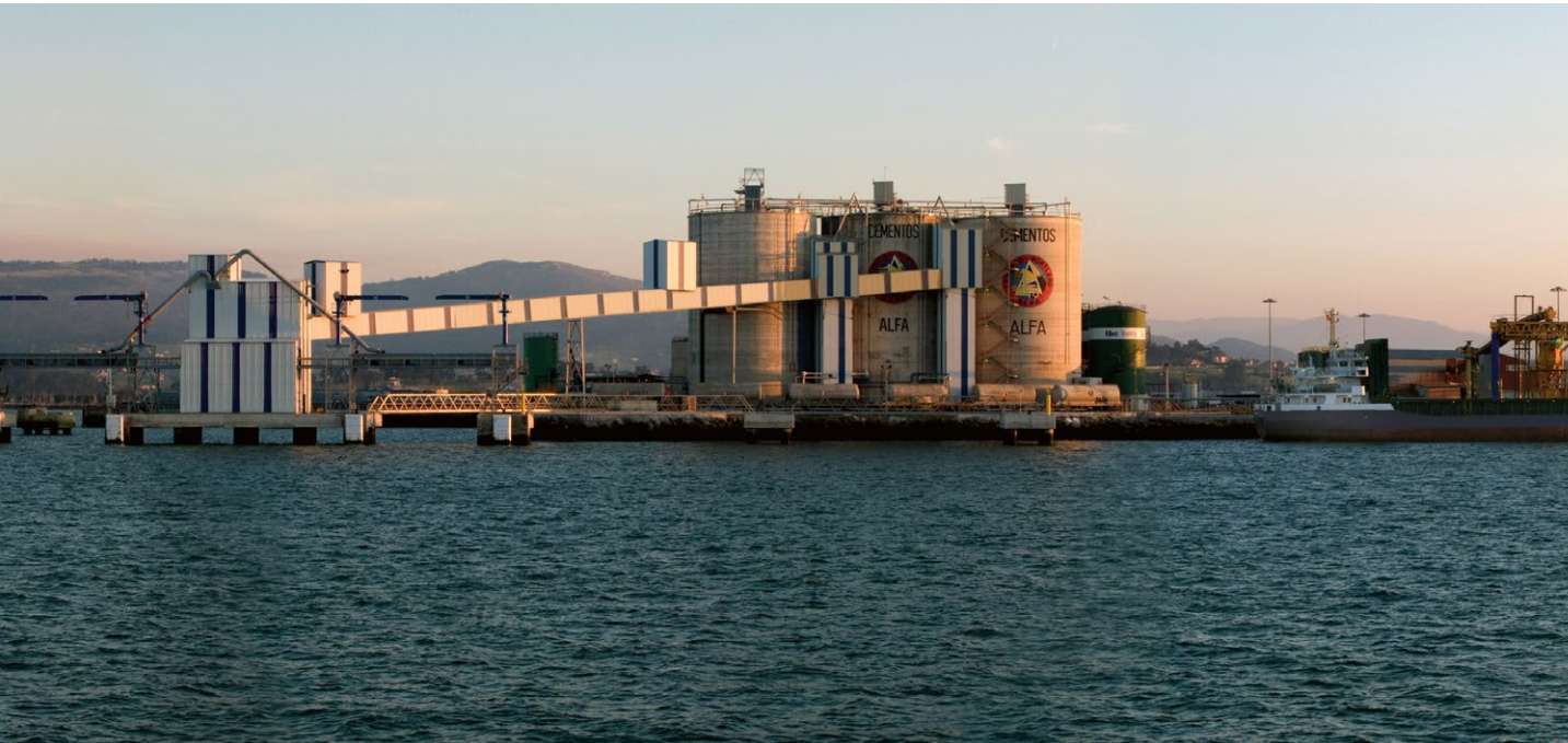
Raos Port Terminal, Santander (Cantabria, Spain).
