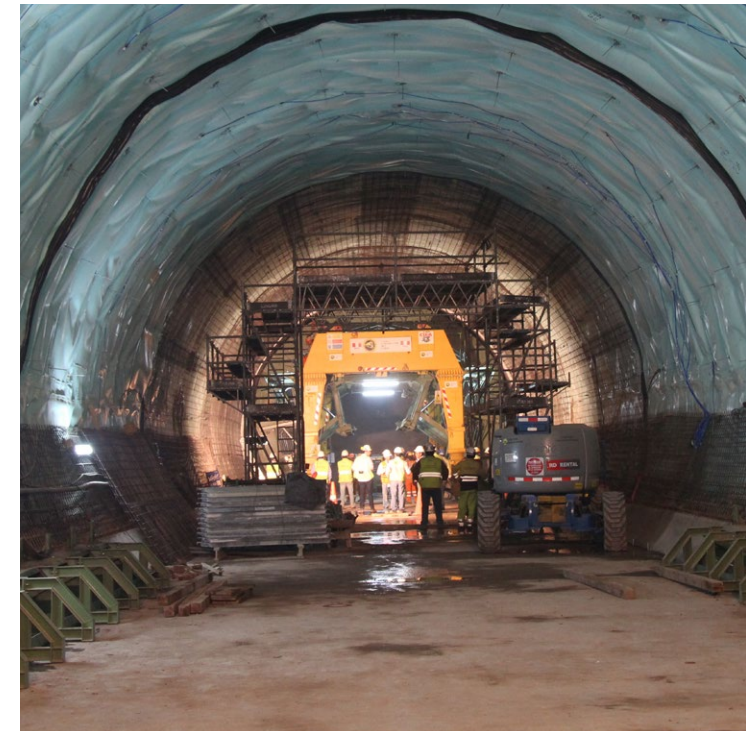
Line 2 and branch line 4 of Lima Metro (Peru).
