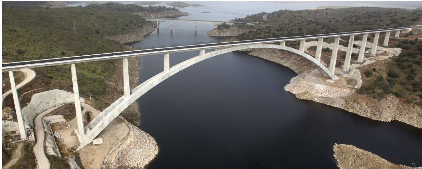
AVE Madrid-Extremadura. Alcántara-Garrovillas reservoir section (Spain).
