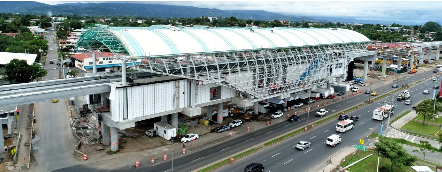
Pedregal Station. Panama Metro line 2.
