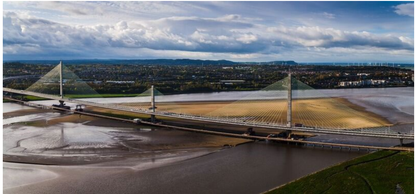
Mersey Gateway Project (United Kingdom).
