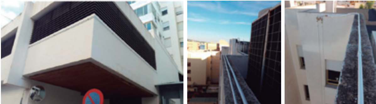
Gas Reception Facility built with Multilayer Systems in Ibiza (Balearic Islands)
