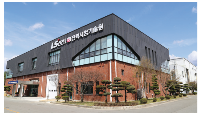
Front view of PT&T
