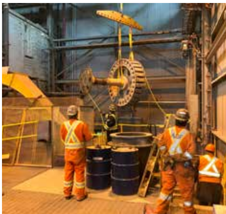
Removing a rotor for refurbishment at the Sigma mill, Lamaque, Canada.
