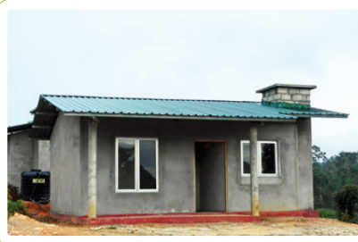
New Houses Logie Estate
