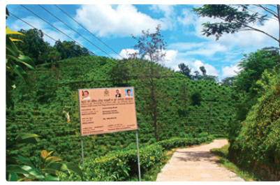
Road Development Deniyaya Estate
