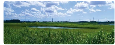
Shibakawa Daiichi Flood Control Reservoir
