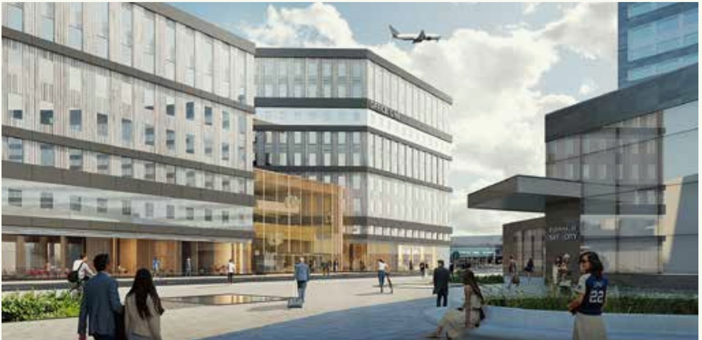
Office One in the new city block under construction at Arlanda Airport.
