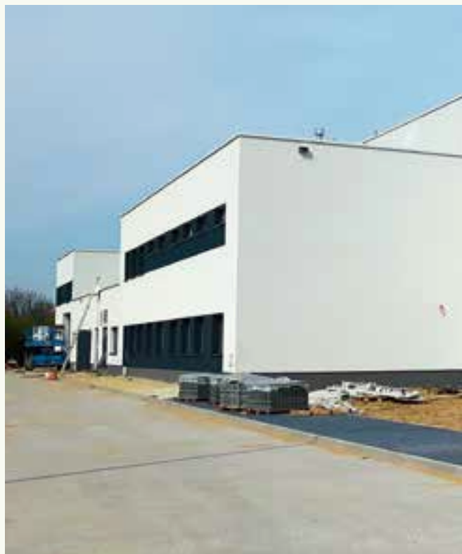
The new paint shop was completed in just eight months.
