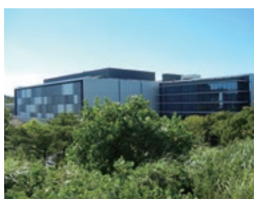
Tokyo Data Center I, boasting advanced environmental performance
