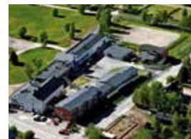
Bojan 2, Haparanda correctional facility
