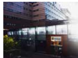
Kronoberg 18, Police Authority's offices
