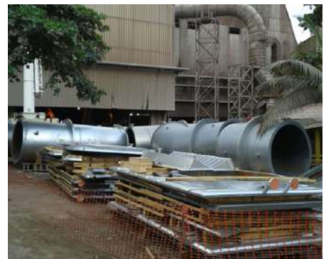
Dedusting installation at Timoteo (the size of 6-floor building) and renovation works in progress with new pipes ready to duct dust.
