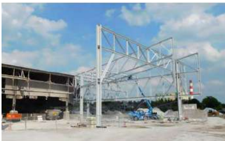
Erecting the building for the "cold" zone of our slag yard at Châtelet in summer 2017.
