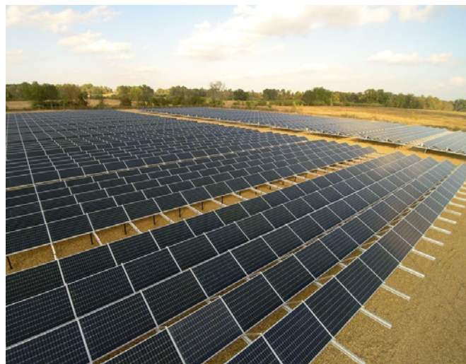
At our Nashville, Arkansas plant in the USA, we built our first solar power generating facility with 1,3 MW capacity. It is expected to reduce our CO 2 footprint by approximately 52,000 tons over its 25-year lifespan.
