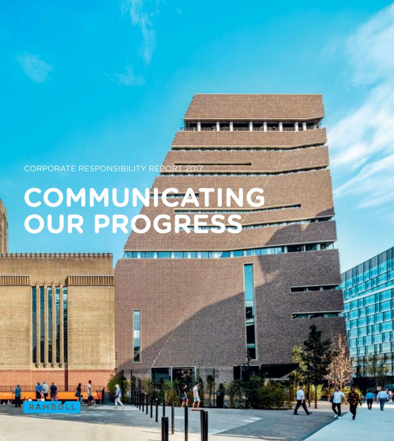
Cover: The iconic Tate Modern extension in London is characterised by its striking façade, made up of 336,000 bricks that were preassembled off-site and carefully chosen to ensure long-term performance. The building's concrete frame uses a solution that has lower CO2, resulting in a lower carbon footprint. Image: Daniel Shearing.
