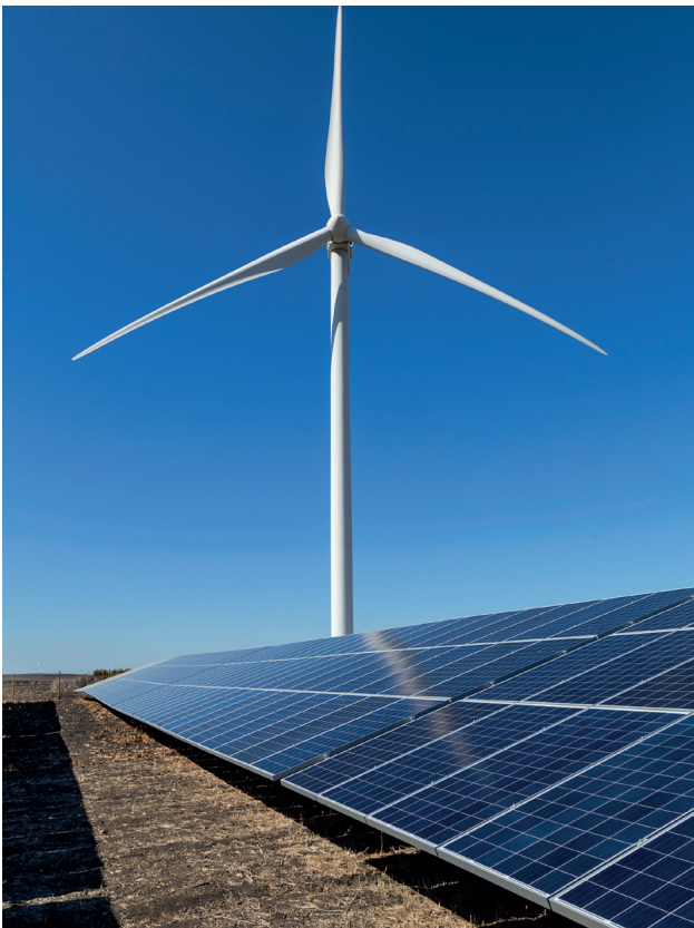
El Conilete hybrid power plant installation
