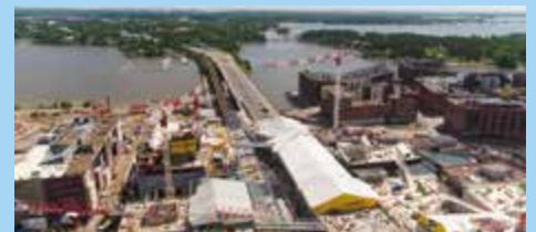
SCAFFOLDING & WEATHER PROTECTION
