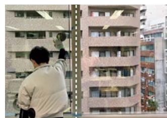
Energy-efficient dual-pane windows installed in the head office At left: with dual panes installed At right: Before dual-pane installation with low-E coating
