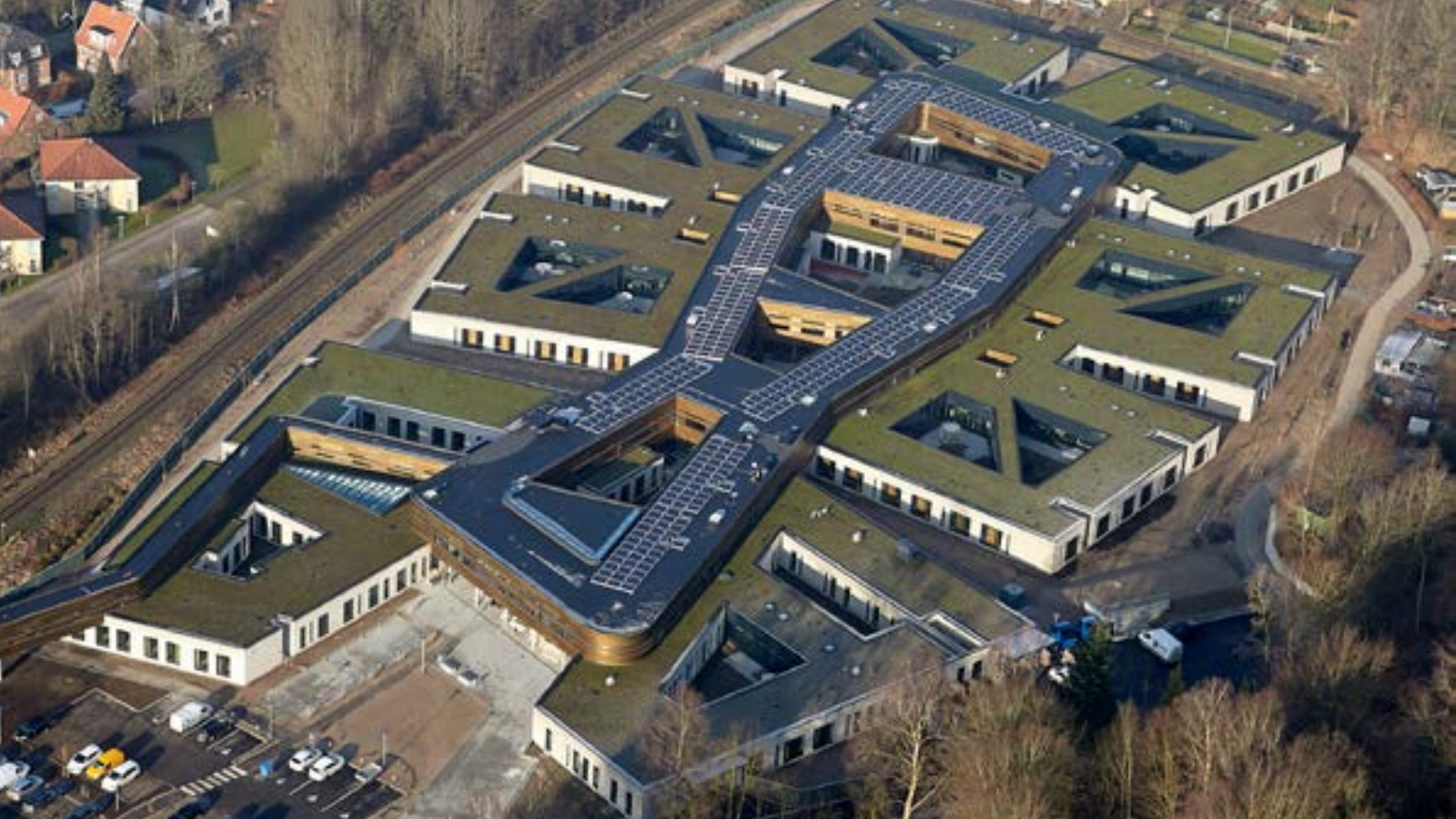
PensionDanmark co-invested in Denmark's first PPP hospital, the psychiatric hospital in Vejle, which was completed in 2017
