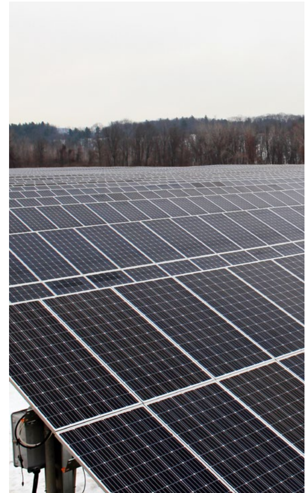
Angled solar panels to shed snow and allow for maximum energy production.
