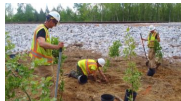
Safety first during restoration.
