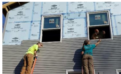
Habitat for Humanity project.
