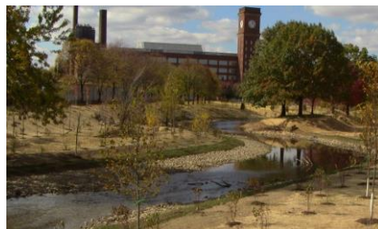
Stream restoration project on Cuyahoga River.
