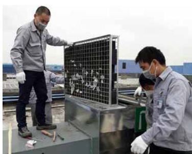
Carbon filter being installed to the outdoor exhaust equipment (China)
