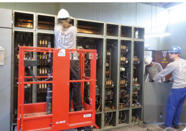
ATS teams are working on the upgrade of the low tension cabins in Ampsin hydro plant (August 2016).
