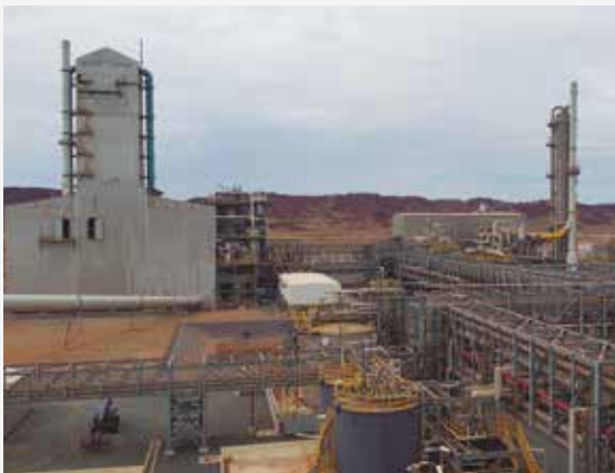
Photo of the project for Yara in Australia, completed in 2016
