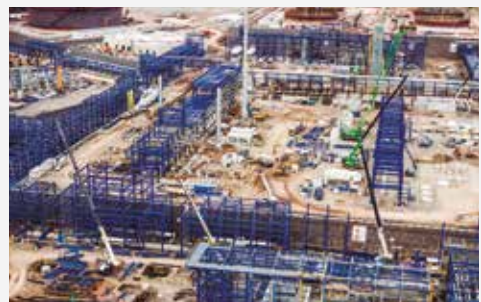
Aerial image of the SOCAR project.
