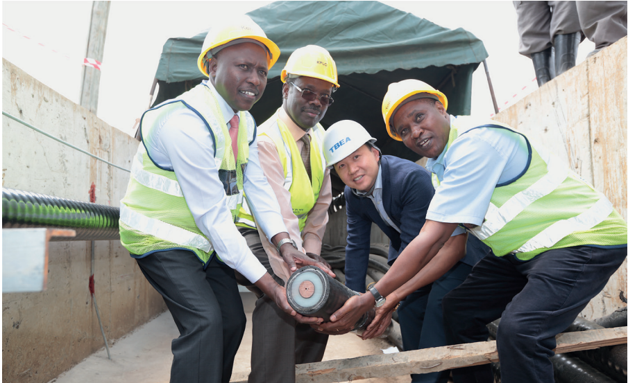
Laying of underground cable at Langata, Nairobi.
