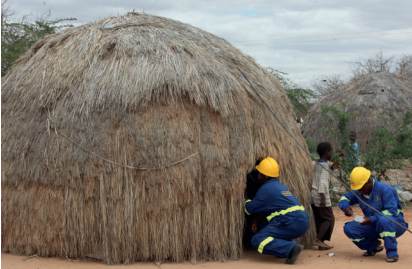
Electrification project in Madogo village, Garissa County.
