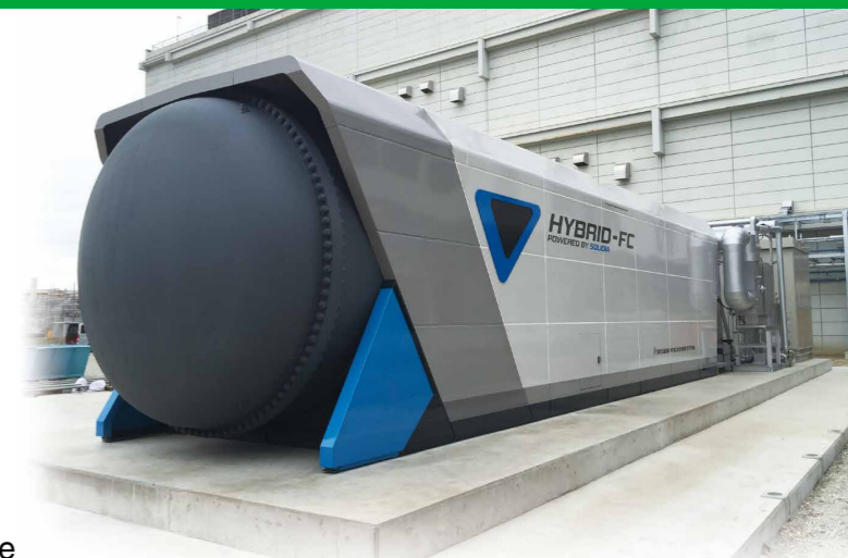
Pressurized hybrid power generation system installed at the Komaki Plant
