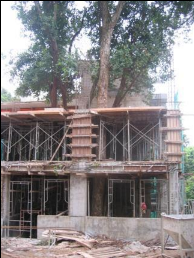
Building on stilts allowed better protection to the trees and to build on a sloped terrain.
