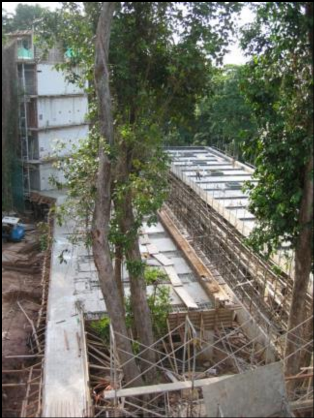
Building on stilts allowed better protection to the trees and to build on a sloped terrain.
