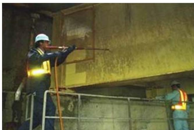
桁端部塩分洗浄状況
