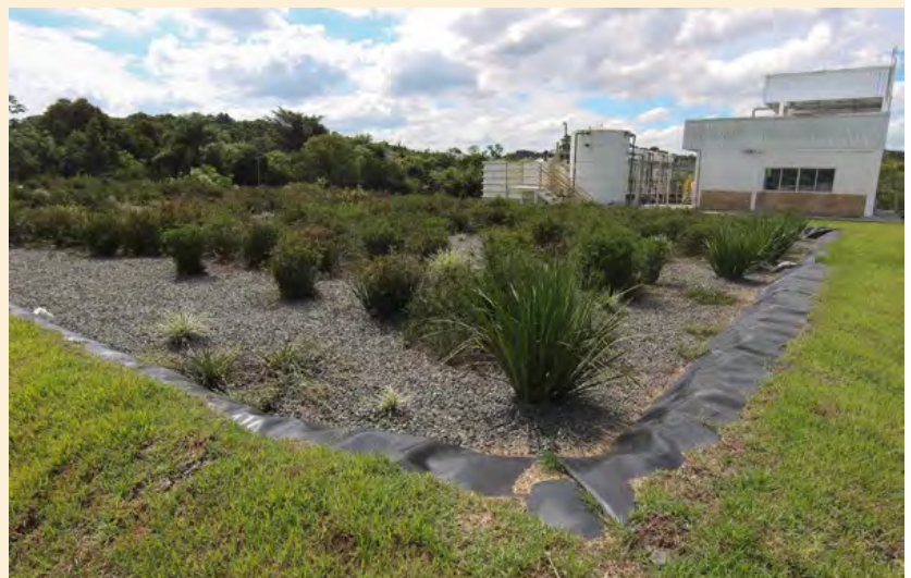
A wastewater treatment facility sits near Joinville Engine’s filtering gardens, where the plants and soil are used to filter wastewater.
