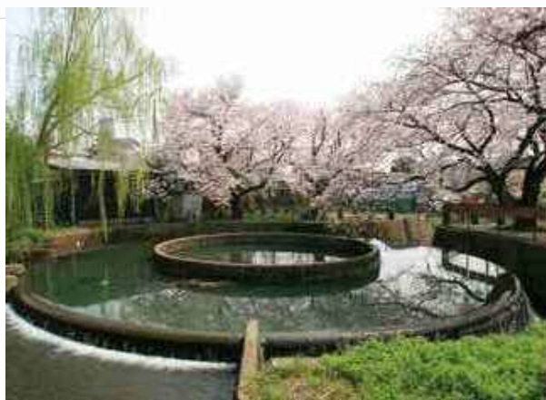
先人の知恵が詰まった国登録有形文化財「ニヶ領用水久地円筒分水」 “Nikaryo Aqueduct Kuji Ento Bunsui”, a cylindrical water division system that is one of the national registered tangible cultural assets
