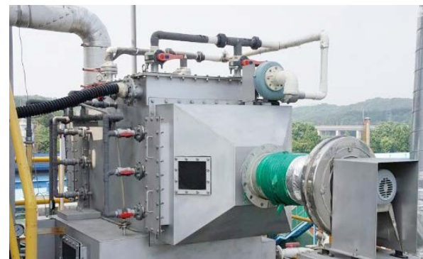
Wet-type Electric Precipitator
