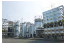
Water treatment facilities installed at a brewery of Asahi Breweries, Ltd. Water reused within the brewery is treated using these facilities.
