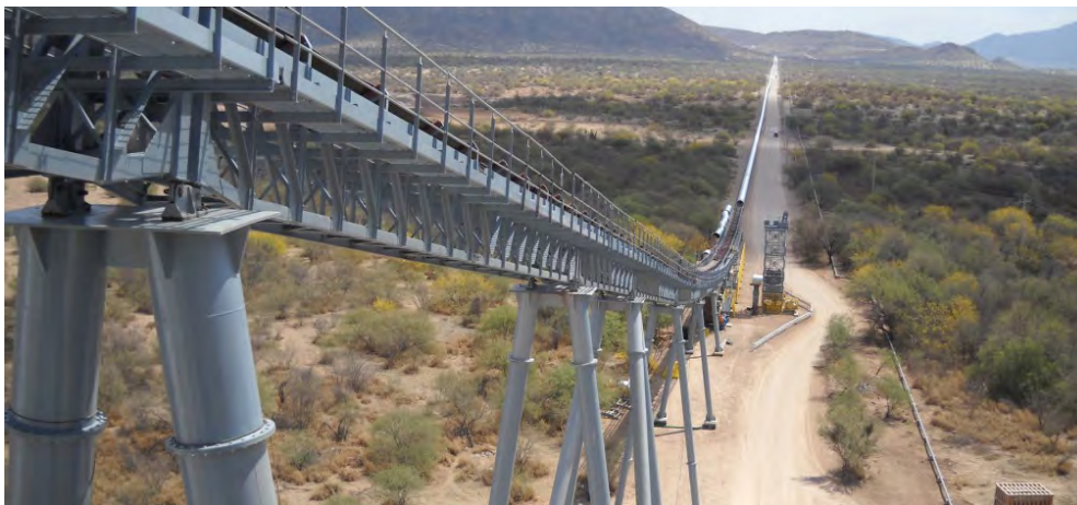
General view of the 4.5 km curve Overland Conveyor in Hermosillo. Mexico.
