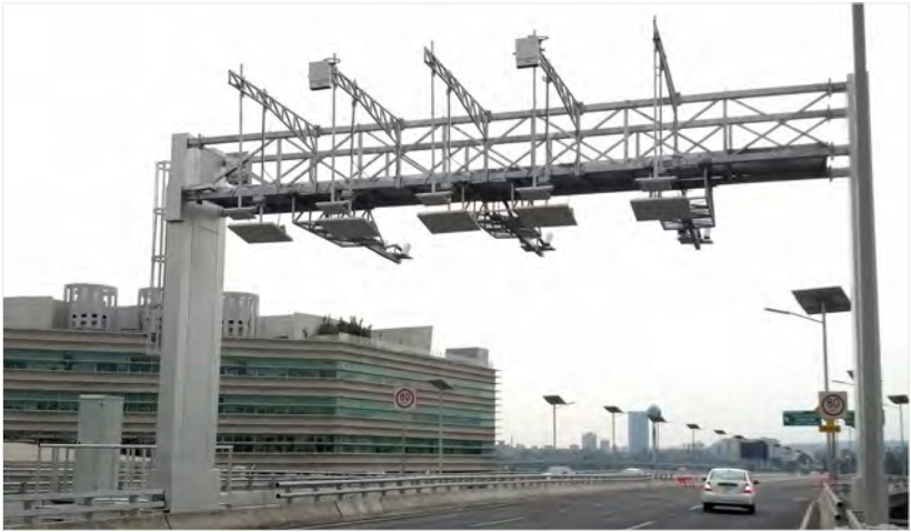
Advanced toll control and management system. Free-flow gantry.
