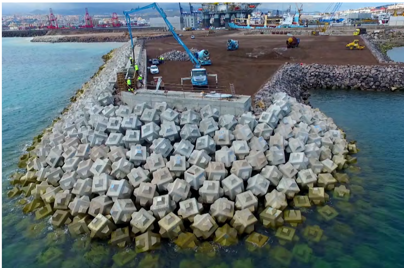
Armor of Cubipods in the Port of A Coruña. Spain.
