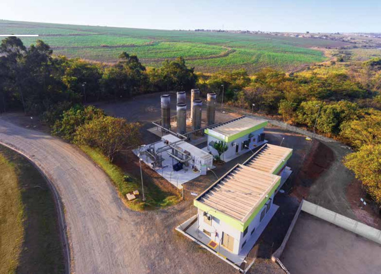
Aerial view of biogas burning facility in Paulínia (SP)
