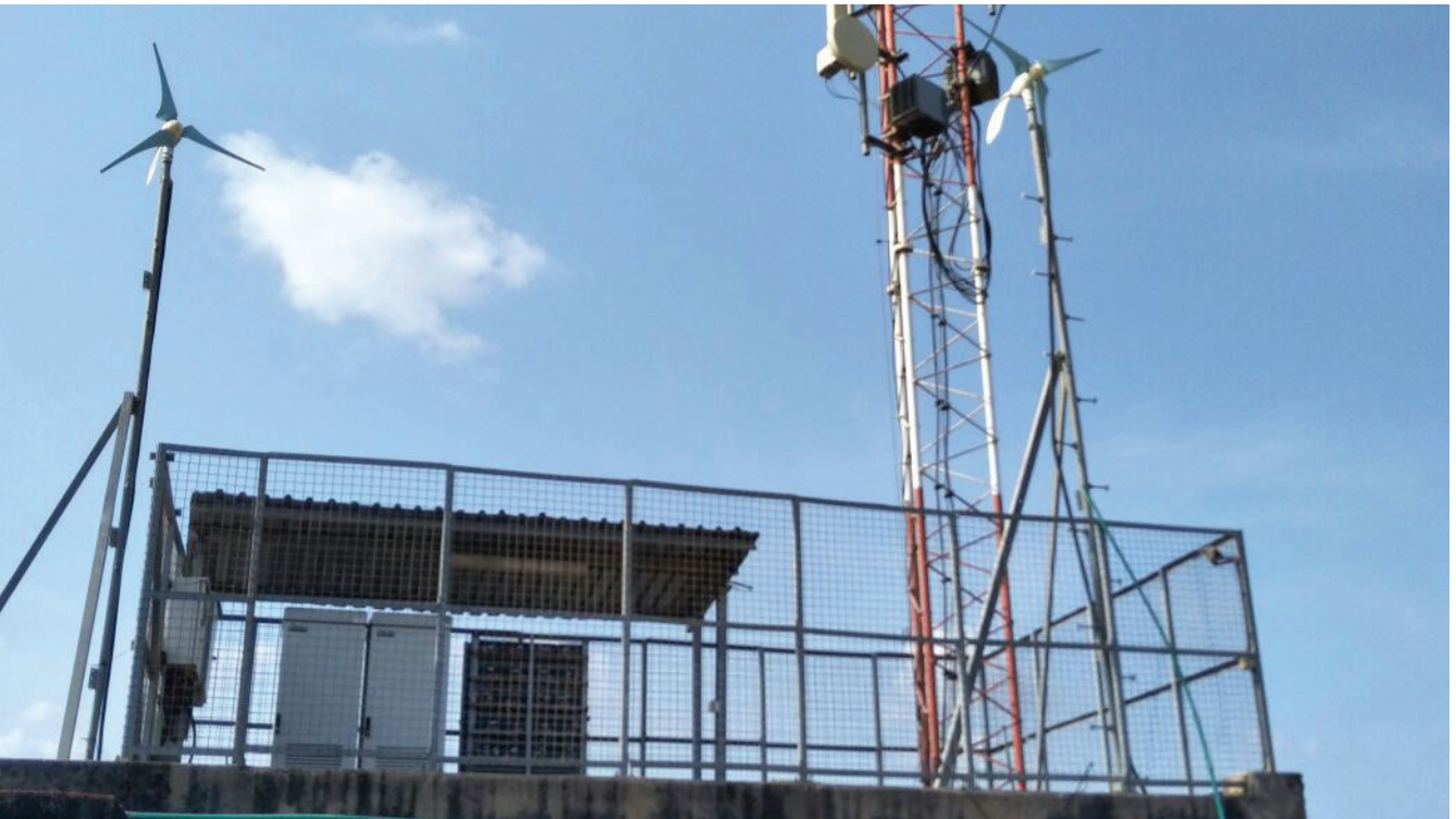
Wind turbine installed by Broadband at a Mombasa site
